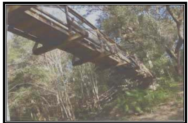
Overhead Bridge (S)
